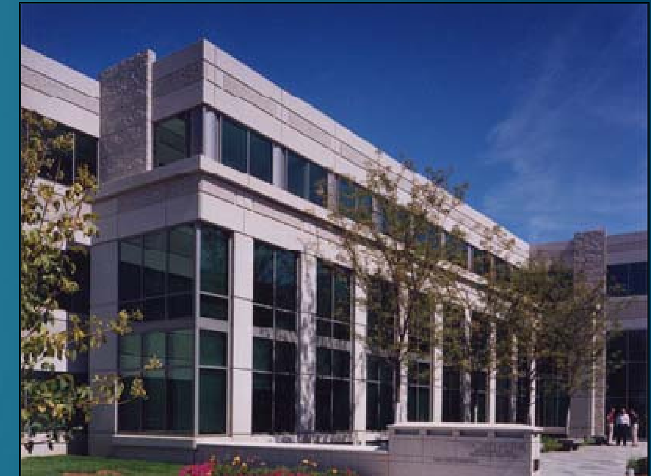
A 179,800 sq. ft., three-story steel frame office building with architectural precast façade
